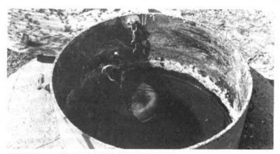
Float-valve regulates water level in stock tank.
